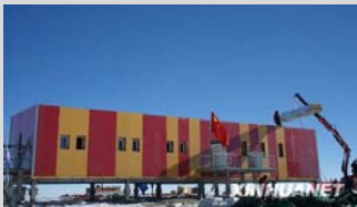
Kunlun Station under construction. Photo courtesy of Xinhua
