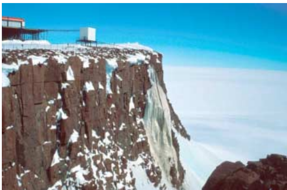
Photo 2: Waste water discharge point at SANAE IV
