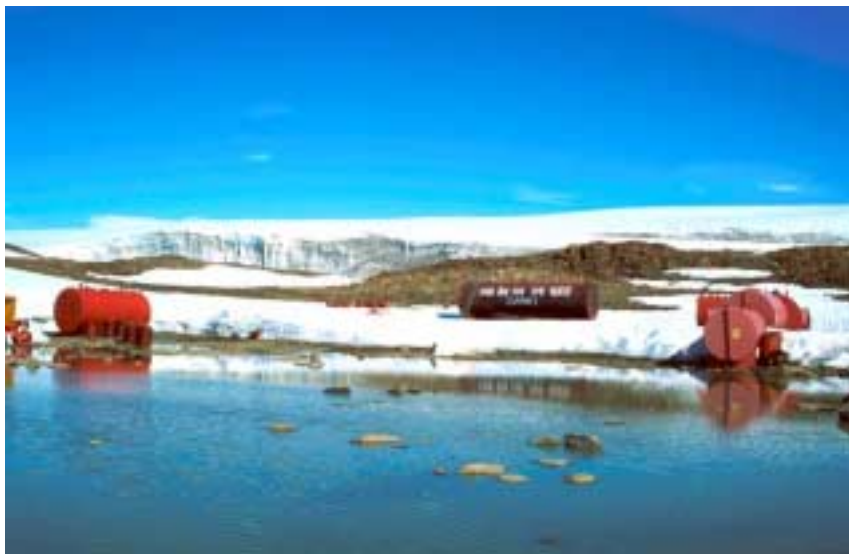
Photo 5: Fuel storage area at Maitri
