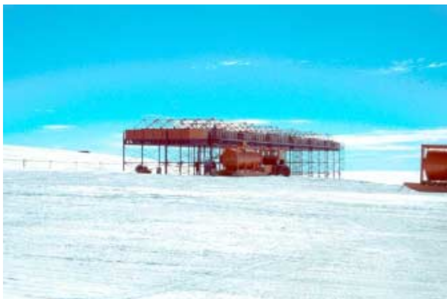
Photo 12: The bulk fuel storage at SANAE IV
